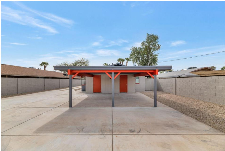
Covered Parking and Storage Rooms
