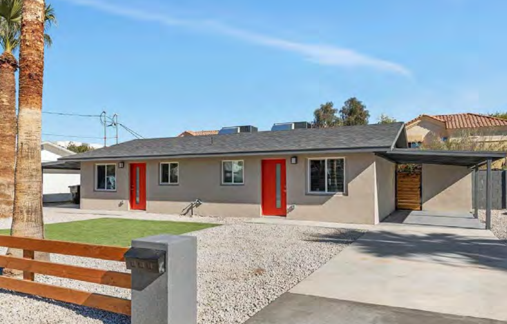
Covered parking & secure gate access to yard
