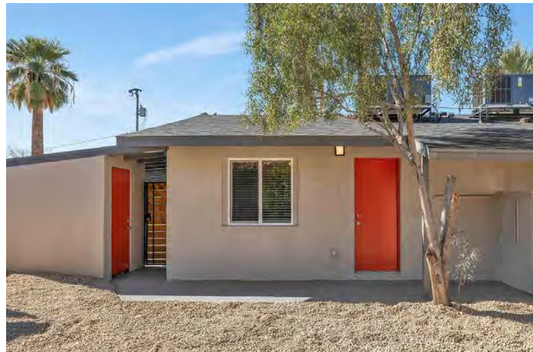
Individual Storage Room
