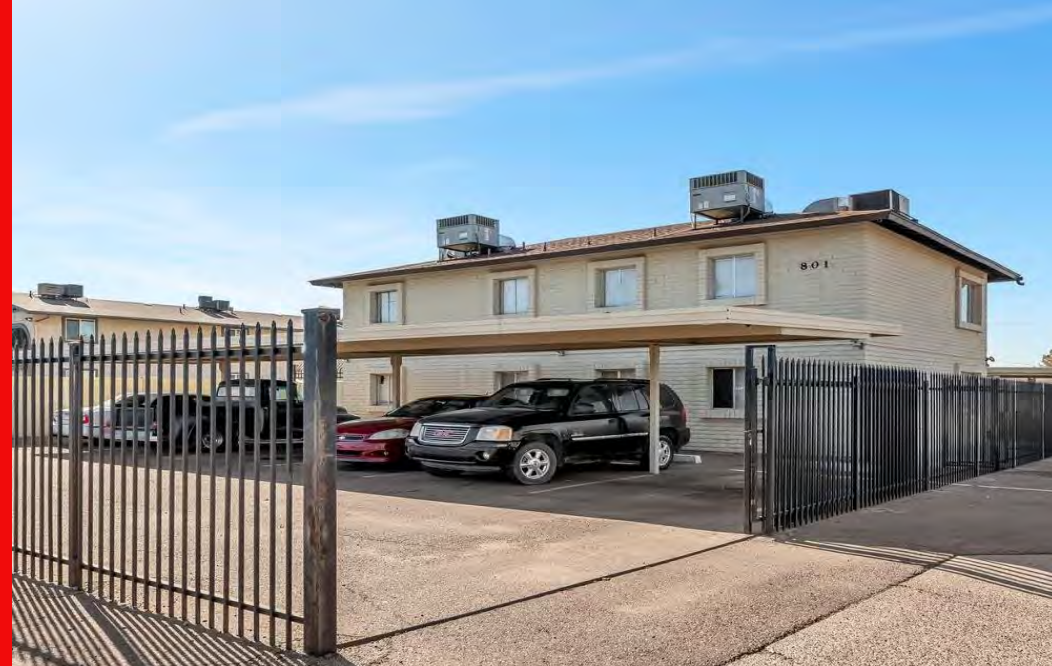
Secure Parking Area
