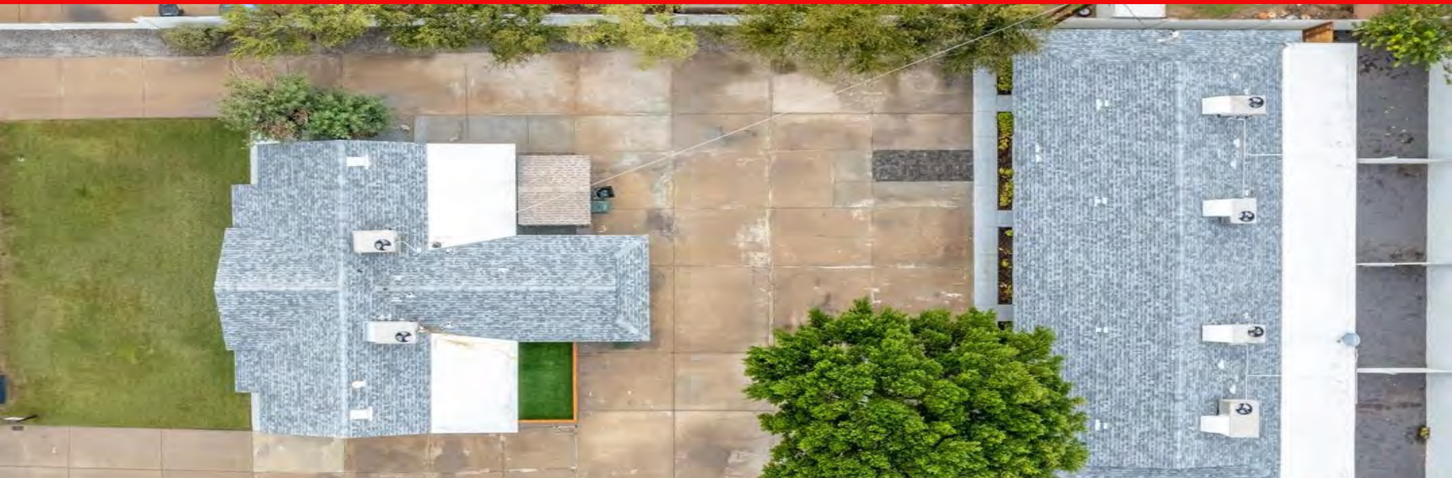
Freshly Landscaped Front Yard & Common Area/Parking
