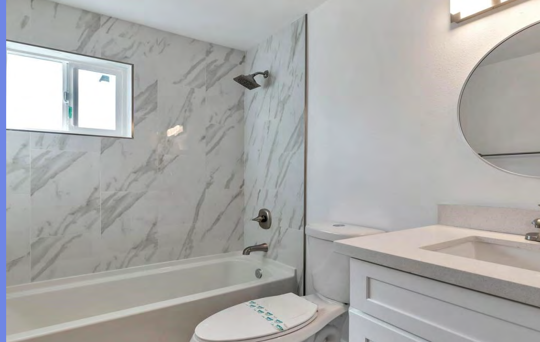
Typical Bathroom Remodeled
