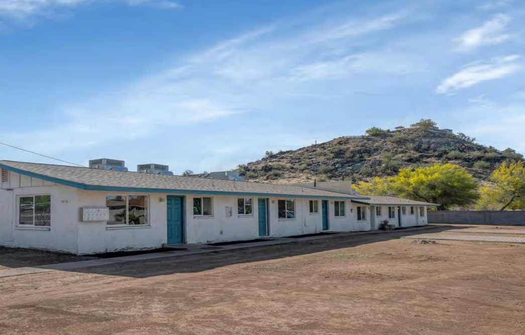
Exterior of Building
