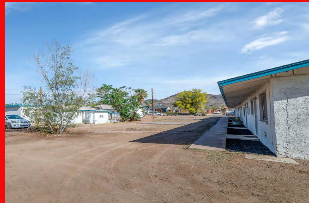
Exterior of Building
