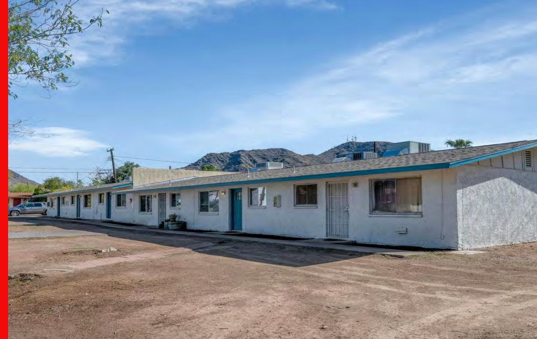
Exterior of Building
