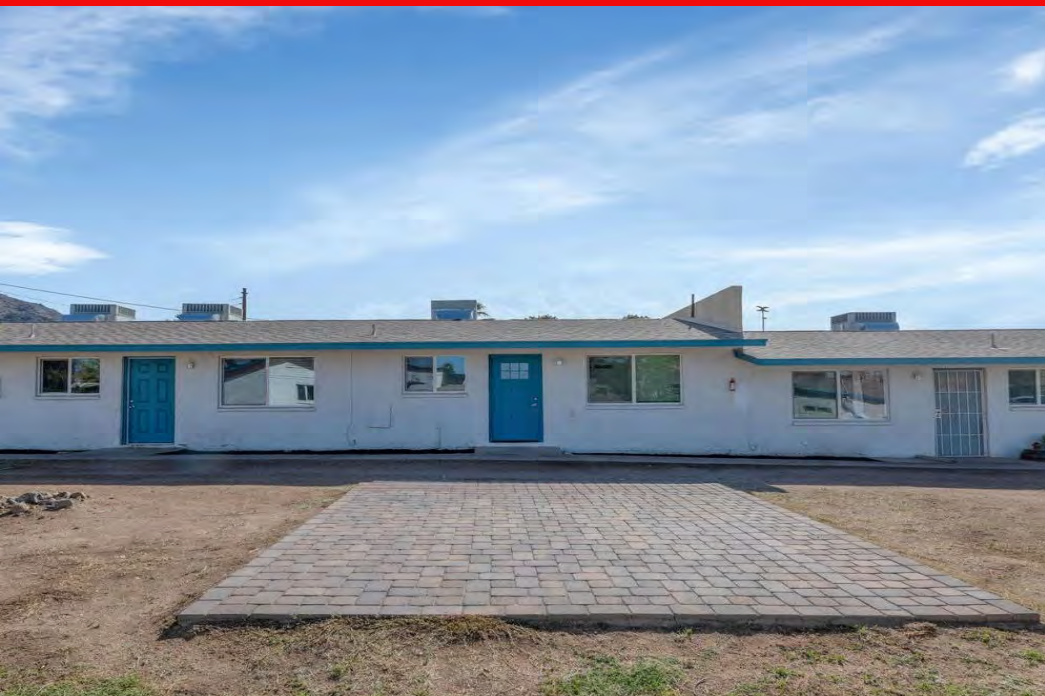
Exterior of Building
