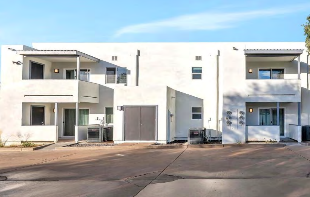
Private Balconies and Storage Rooms
