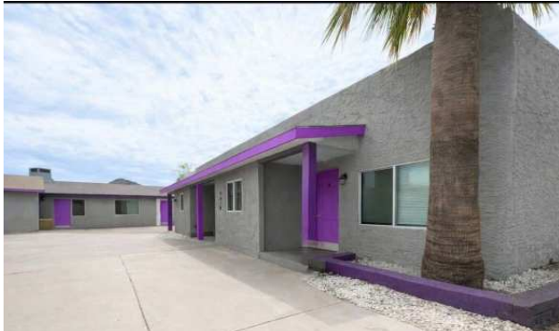
GATED PAVER COURTYARD
